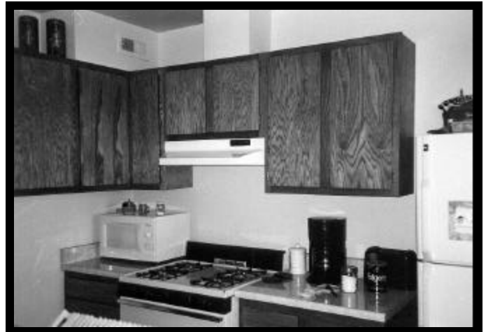
Totally refurbished kitchens were part of the rehab work
