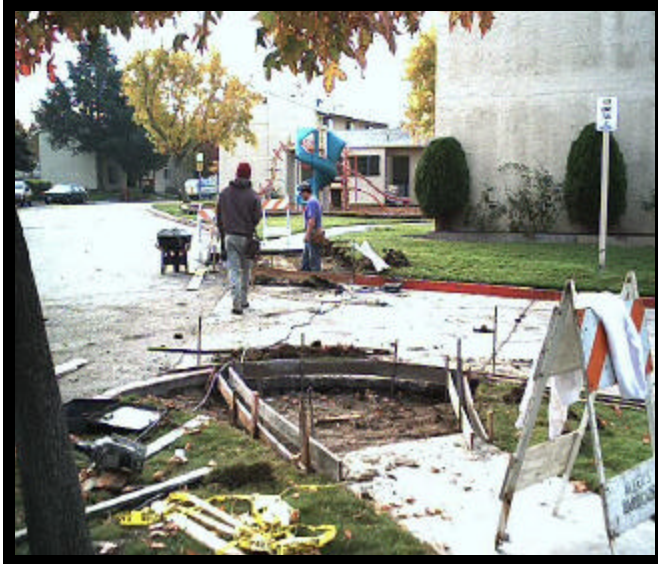
Cutting curbs was part of making property completely accessible to disabled persons.
