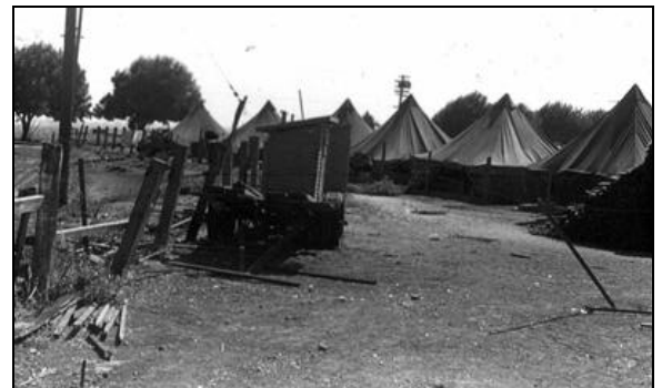
Farm worker housing conditions like these above are examples of why Dolores Huerta, Walter Ruether, and Cesar Chavez founded the NFWSC.
